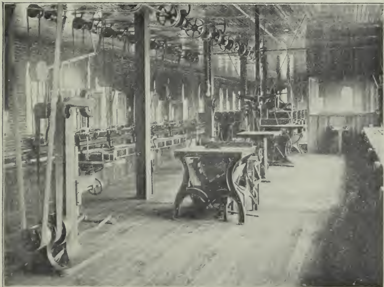
Wood Working Room Looking East.
